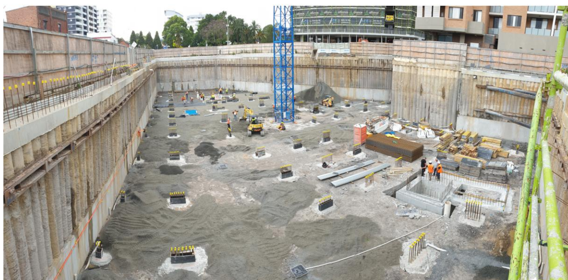
Figure G8 Real excavation and support – Project in Lidcombe 2019
