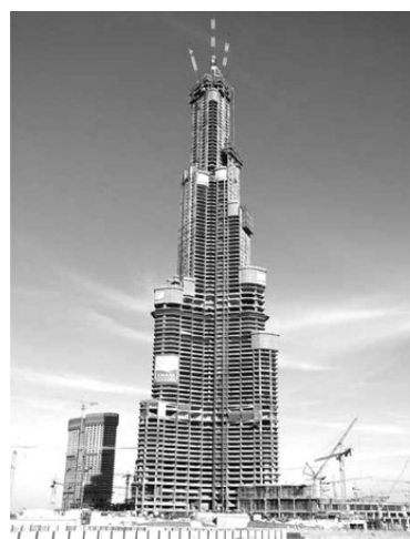
Fig. 2—Construction photo of tower.
